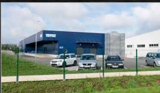
7. 12. In 2021, a new hall with a usable area of almost 3,000 m 2 was approved.
